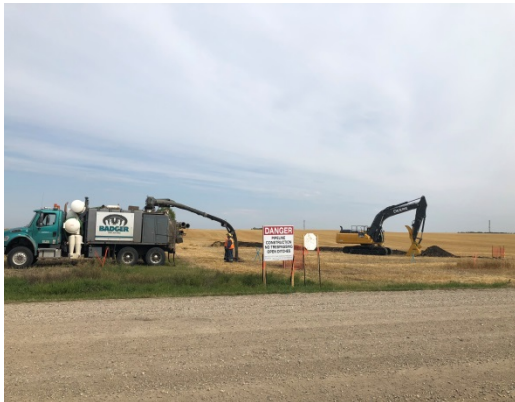
SF 38, photo facing north, hydrovacating taking place and topsoil being stripped by excavator.
