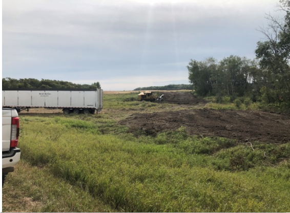
SF 38, photo facing south east, mulching taking place.
