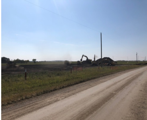
SF 35, south side, photo facing west, ROW being stripped.
