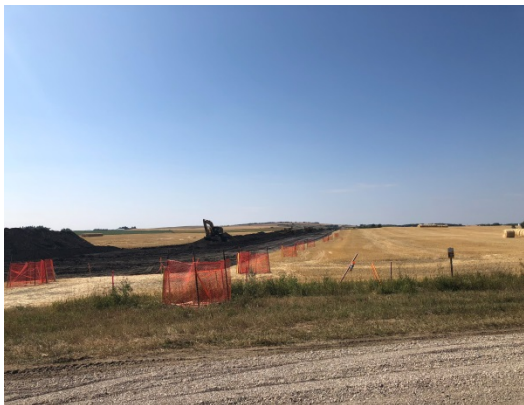
SF 34, photo facing west, topsoil being stripped and pushed by multiple dozers.
