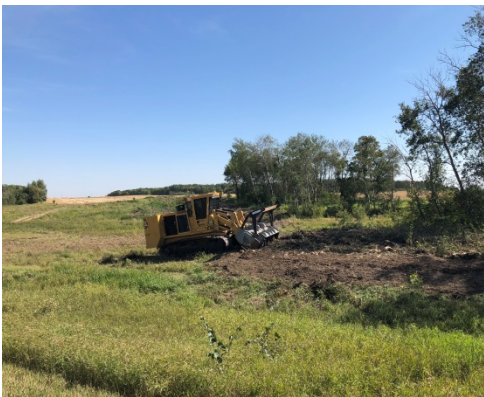
SF 38, photo facing north east, mulching taking place.
