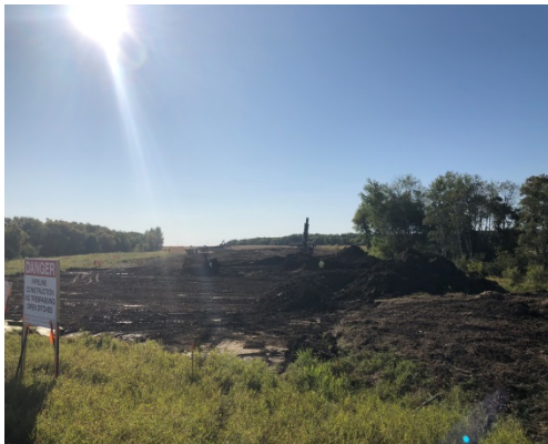
SF 38, south side, photo facing south east, excavator and dozer pushing dirt.
