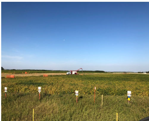
SF 41A, photo facing west, one hydrovac just doing what a hydrovac does.
