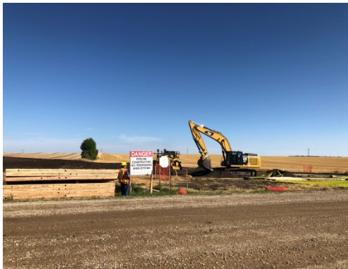
SF 38, north side, photo facing north excavator and dozer pushing topsoil.
