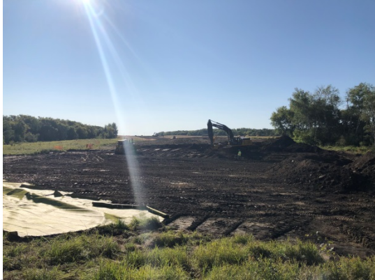
SF 38, south side, phot facing east, another photo of the equipment pushing dirt.
