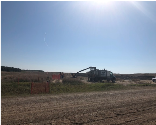
SF 36, photo facing east, badger hydro vac just hydrovacating.
